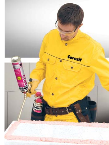
Fixing EPS board in thermal insulation system
