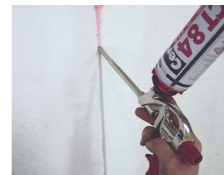
Filling in gaps between boards
