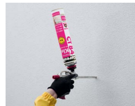
Filling in case of keying panels
