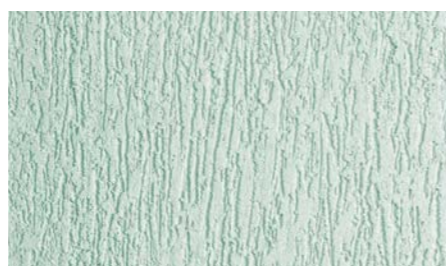
Rustic texture produced with Ceresit CT 35 mineral plaster, grain size 3.5 mm, obtained by floating with a plastic float in one direction
